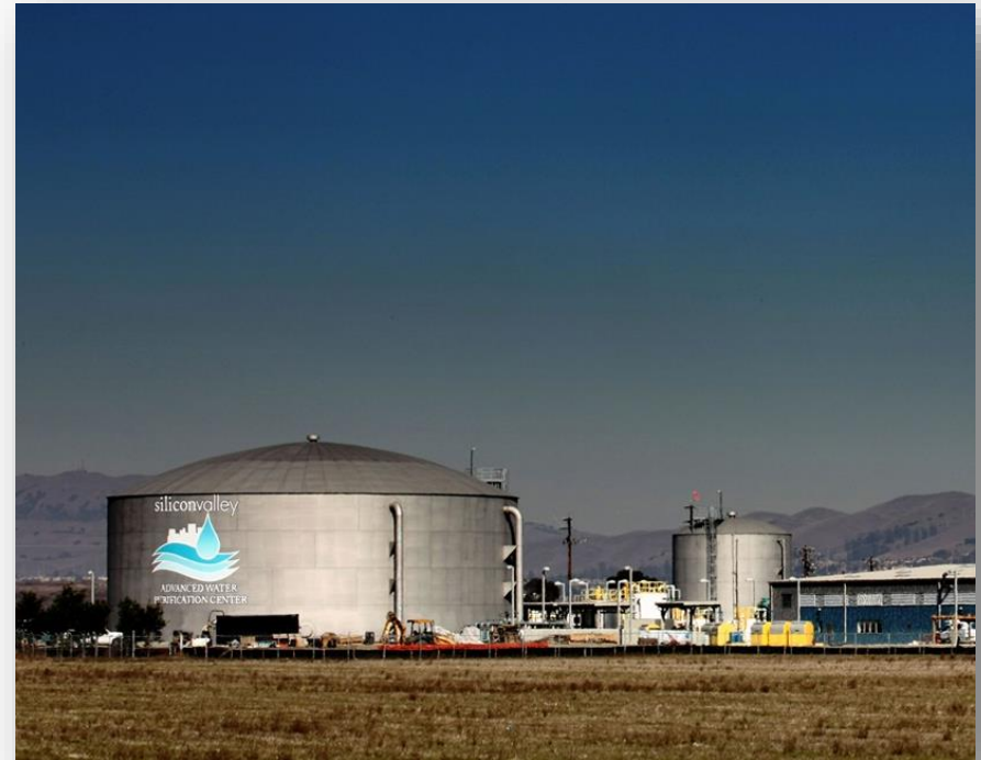
Silicon Valley Advanced Water Purification Center
