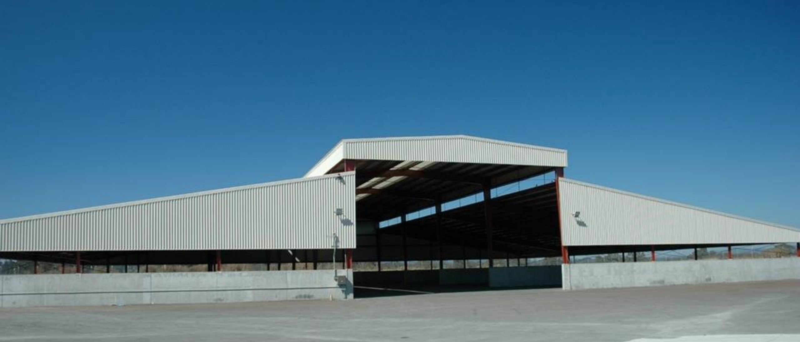
ALPHA Biosolids Storage Facility 7,000 Wet Tons Capacity
