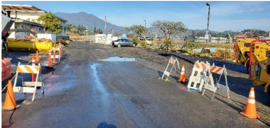
Beginning of Drainage Backflow
