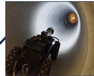
CCTV Target: Single Pipe
