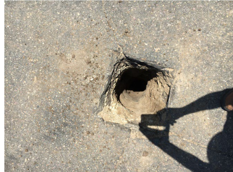
Excavated Hole (to pipe bedding)
